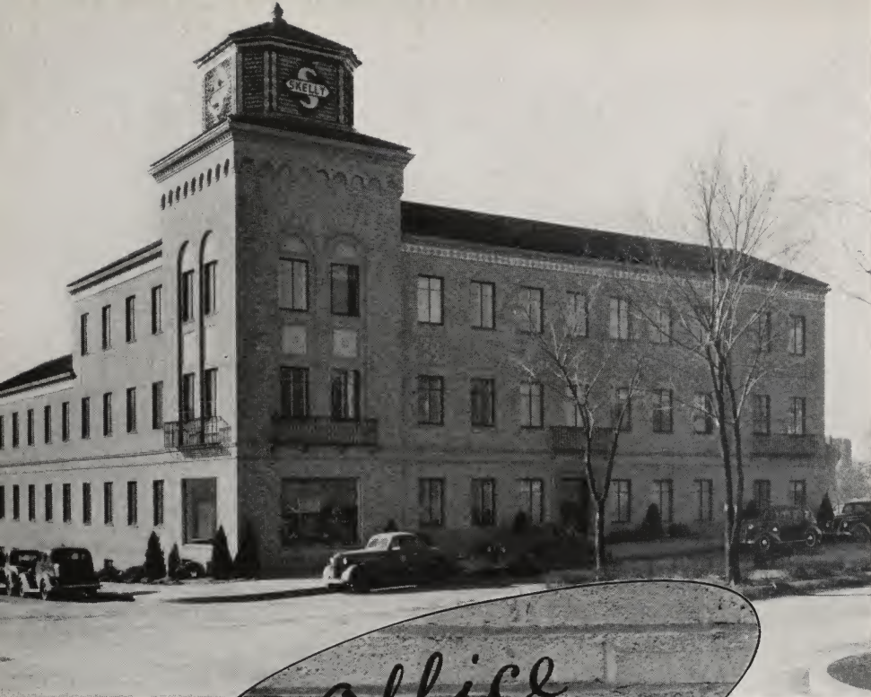
Left —Lightweight concrete masonry backup was used in this modern office building of Skelly Oil Co., Kansas City, Missouri. Edward W. Tanner, architect. J. C. Nichols, builder.
